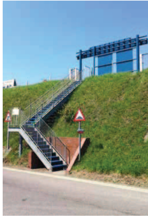
Basin North Road
